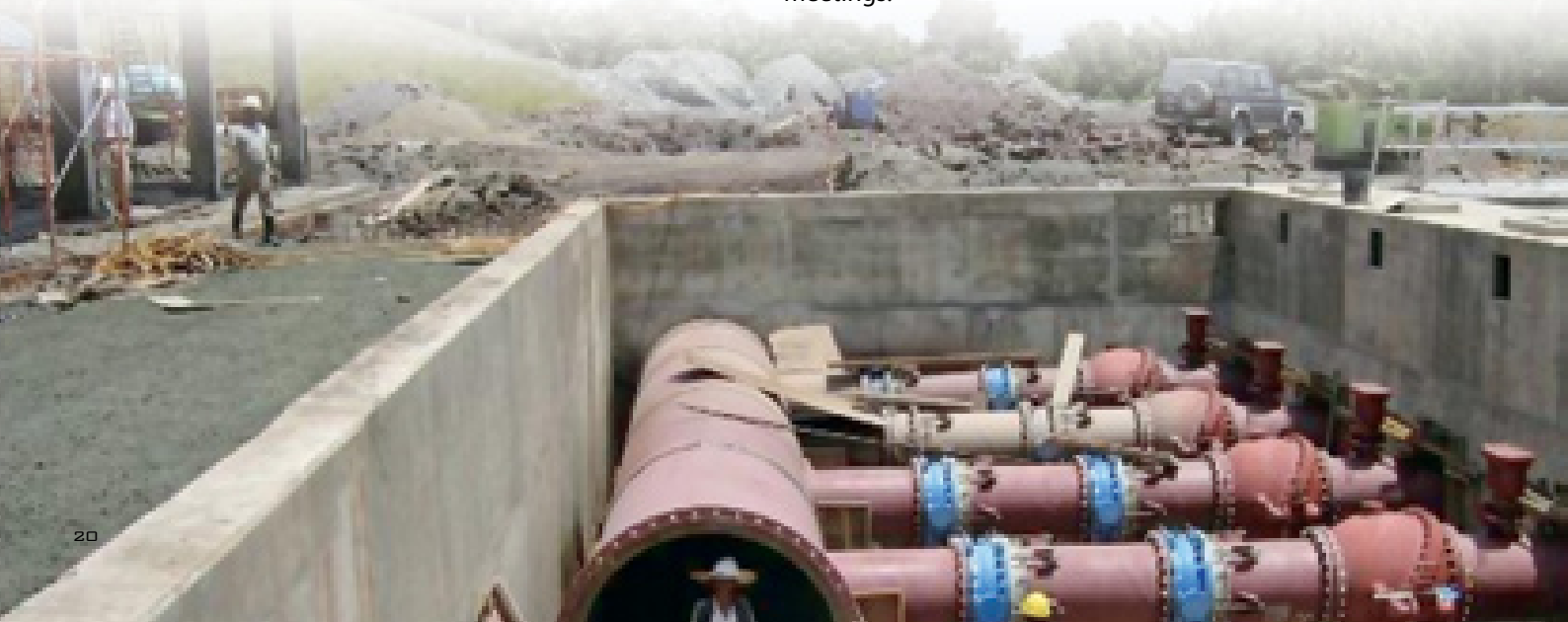
1900 dia Raw Water Manifold Installation - Sandakan
