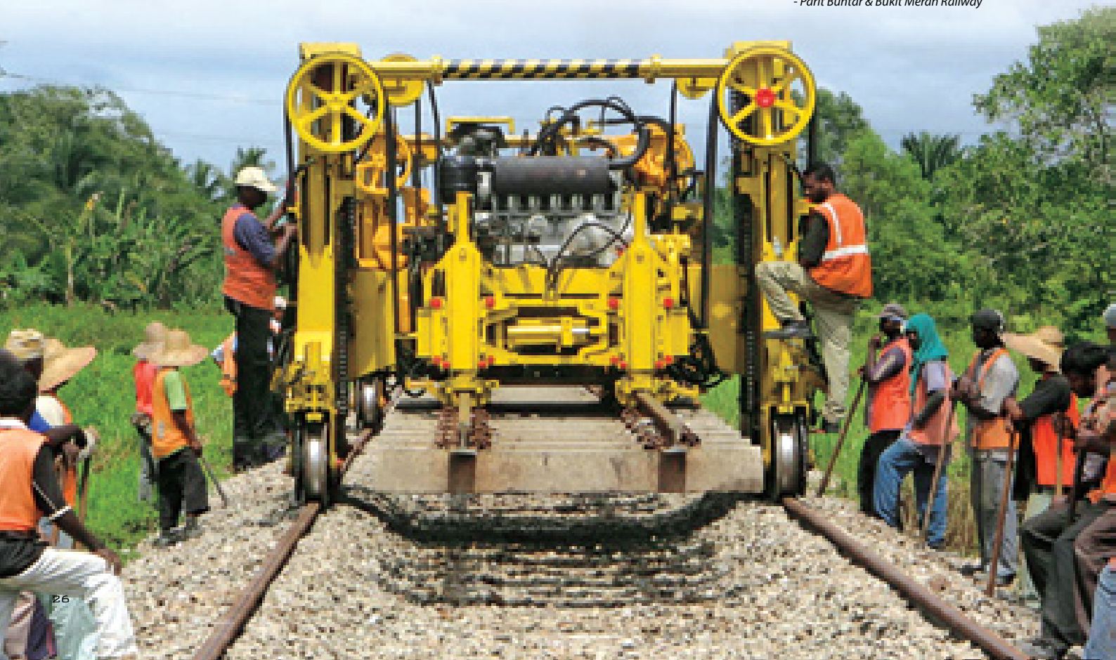
PQRS gantries picking up existing concrete sleeper panels - Parit Buntar & Bukit Merah Railway
